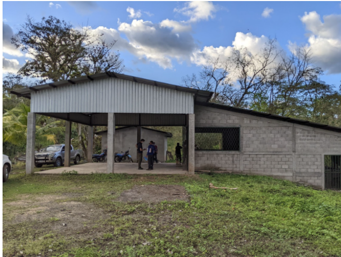
Nicaragua, Tierra Nueva (Agricultural Processing Facility/Building)
